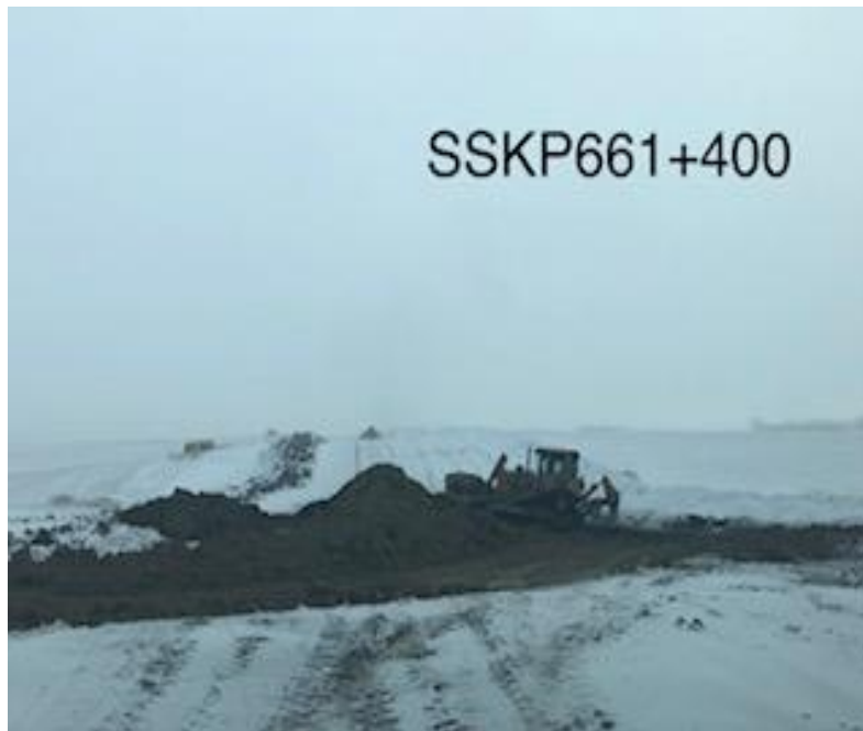
Machine clean up SF73 east
