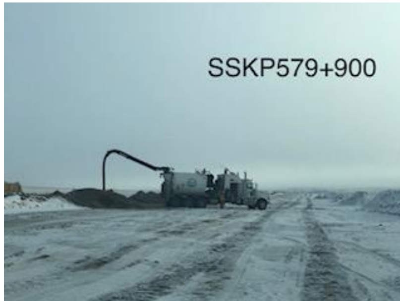
Hydro Vac daylighting SF24 east
