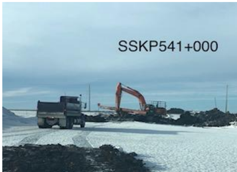
Ramp access removal SF6 east
