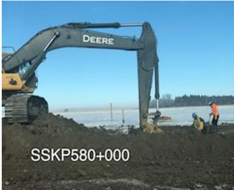
Ovality site – excavation
